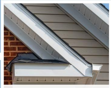
**STEP 6** Apply a drip edge to prevent water from getting to the decking.
