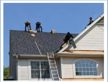
**STEP 7** Install asphalt shingles, beginning with a starter strip to protect seams.
