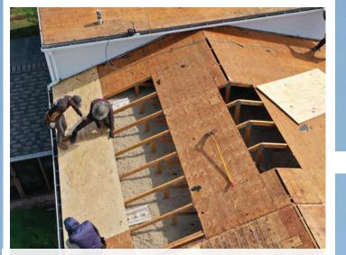
**STEP 4** Inspect roof decking and replace any decking boards that are rotten or soft.
