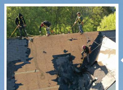
**STEP 3** Tear off the old roof, including flashing, shingles, and underlayments.
