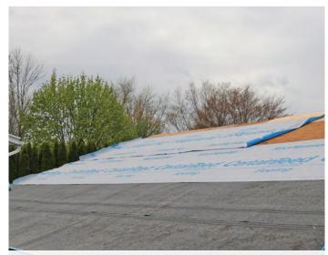
**STEP 5** Install roof deck protection to prevent ice dams and water damage from rain.
